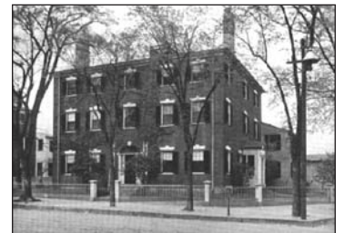
Wourt-Stone House (c. 1805) 132 State Street
