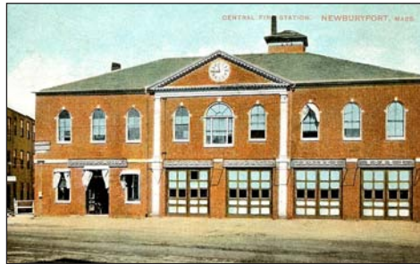
Firehouse (1823), Market Sq. Originally a market building, it was the central firehouse 1864-1980. Theatre & restaurant since 1990.
